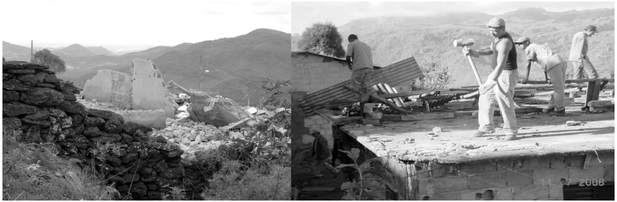
Figures 8, 9. Demolition of irregular constructions; (IPHAN archives, Ouro Preto, MG, Brazil)
