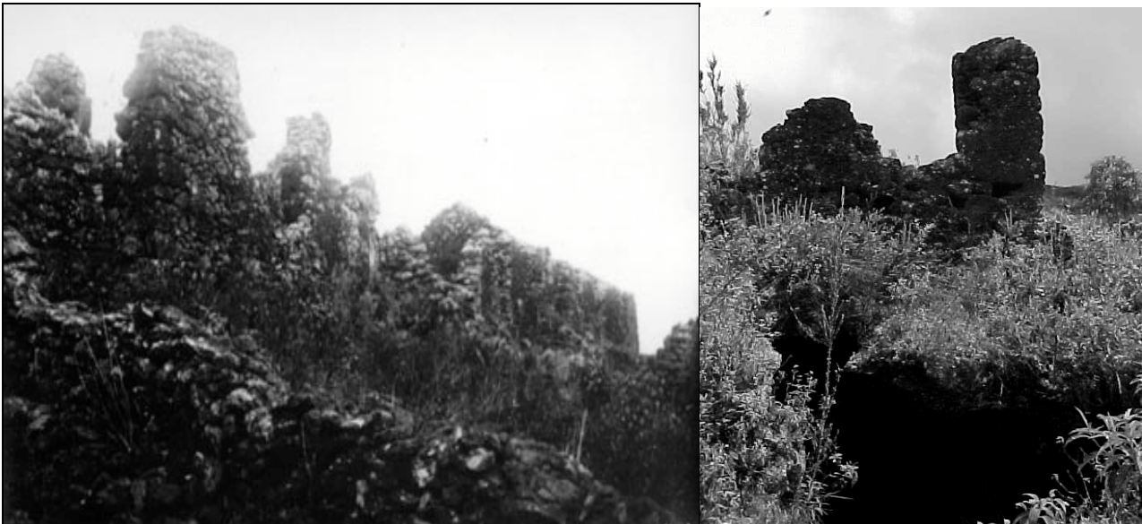
Figures 2, 3. View of the ruins on Morro do Queimada, in the mid 20thcentury (left); (Photo from Luiz Fontana IFAC archives, Ouro Preto, MG, Brazil) and view of part of the ruins at Morro da Queimada(right); (IPHAN archives, Ouro Preto, MG, Brazil).
